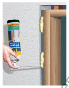
TEKAPUR PU - foam Two component does not require air humidity for hardening.
